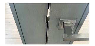
The diagram on the left displays our square edge double doors and the image on the right is how the doors look in situ. At TP Firedoors we do not offer rebated edges to our fire doors, therefore our fire doors offer a quality & contemporary design, provided with closers and fire seals between doors to ensure that doors are correctly protected in the event of a fire.
